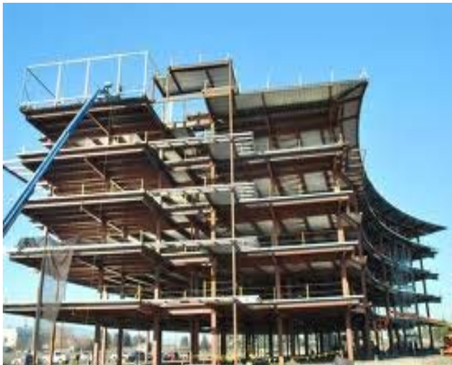
1. Structural Frame System
